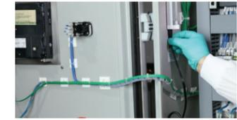
8. Measure from the edges of the control panel to the safety switch on the unit, and mark equivalent measurements on the inside of the control panel door, where the door safety switch will be positioned. If an exact alignment between the two is not possible with your control panel door's structure, you may position the door safety switch so at least ½" of it aligns with the main unit switch.
