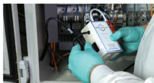
6. Remove the film from the mounting tape on the bottom of the main unit, then place the unit into position and apply gentle pressure for 30 seconds. Repeat this process with the UV-C bulb.
