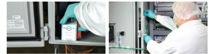
7. Connect the bulb to the main EPIC Panel Sterilight unit using the provided bulb power cable.
