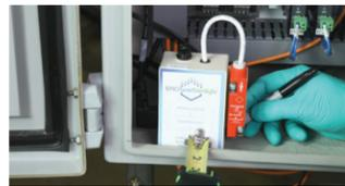
4. Locate a suitable power source within your control panel—either via outlet or direct wire. Then, with the control panel power off, make the electrical connection to the control panel power source.
